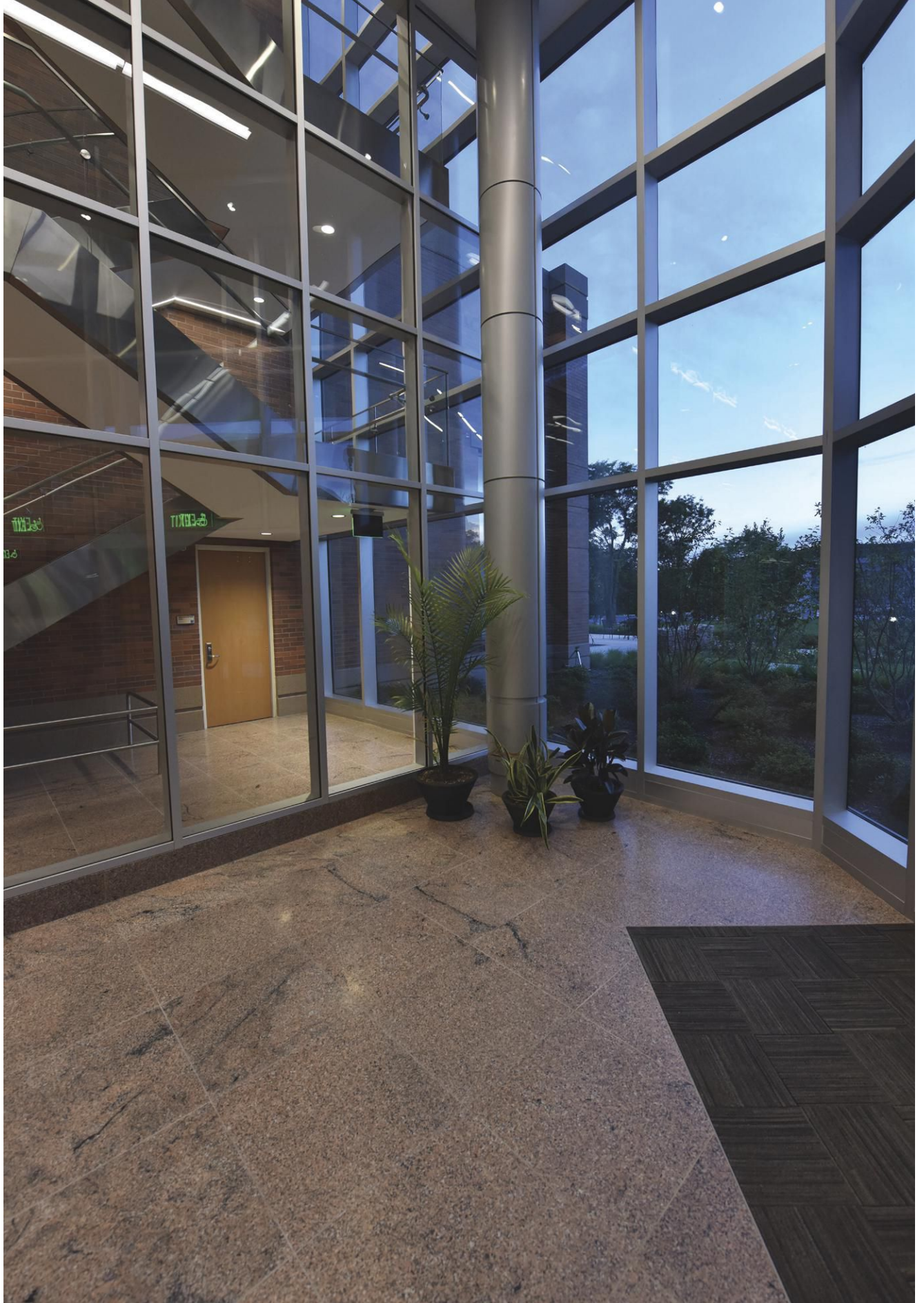
The floor pieces, which were all custom cut — each measuring 2 x 2 x 1½ inches thick — by A. Lacroix Granit of Saint-Sébastien, Quebec, Canada, have a honed finish.
