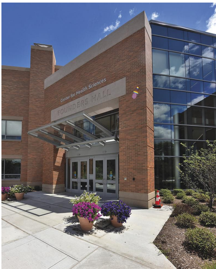
On the outside of Founders Hall, Stony Creek granite was employed for the base course.
